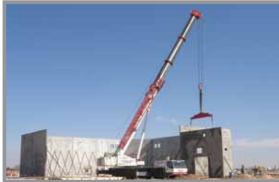
Hermosa Church of Christ: Walls are being erected for the new home of Hermosa Drive Church of Christ in Artesia. Construction is expected to be complete in October 2014.
