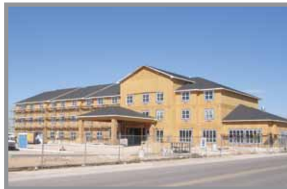
Comfort Inn & Suites: On the corner of Main and 26th Street in Artesia, this hotel will have 66 rooms when construction is complete in April 2014.
