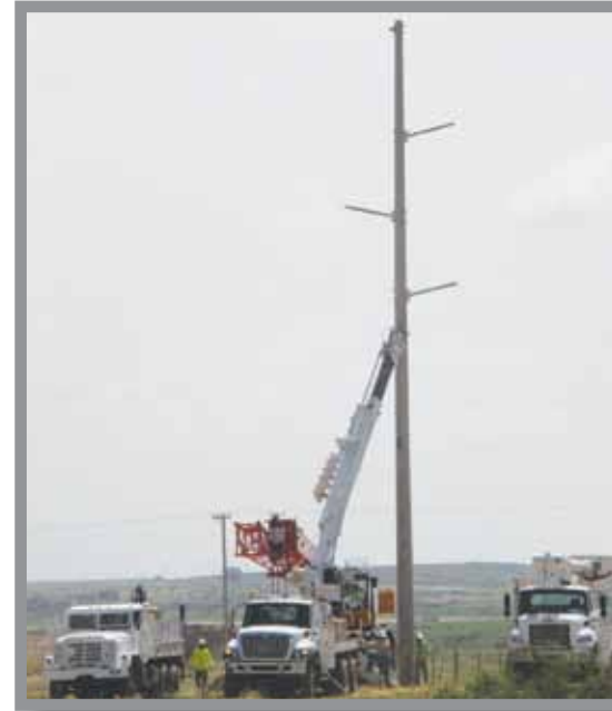
Transmission pole being set North of Roswell.
