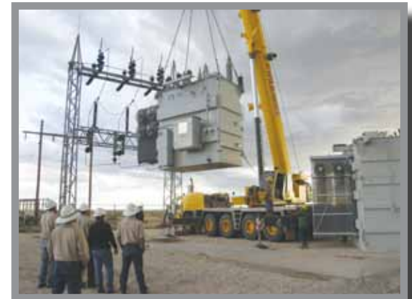
Transformer being set at the ABO substation.
