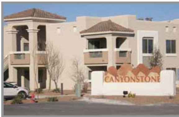
Canyonstone Apartments: When construction is complete at the end of 2014, this apartment complex will have 186 units.
